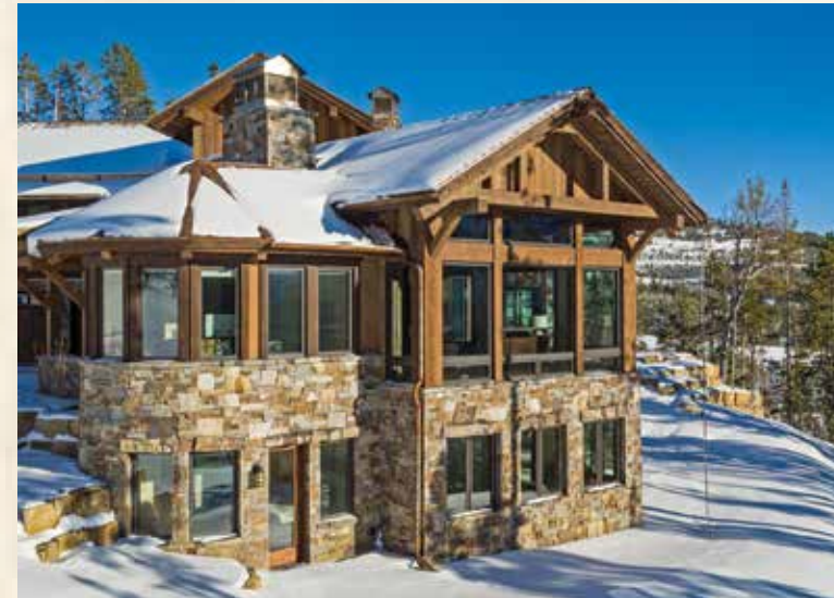
RIGHT: The owners wanted the home to feel as though it belonged in the environment, and used large timber beams and exterior stone to help tie it into the hillside. BELOW: Mountain views drove the layout of key areas of the house.
